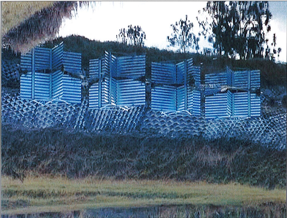
Canal 5 Anti Vortex Replaced
